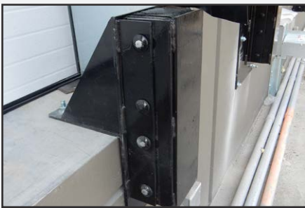
Vertical steel-faced bumpers with gusseted bracket and load distribution plate.
